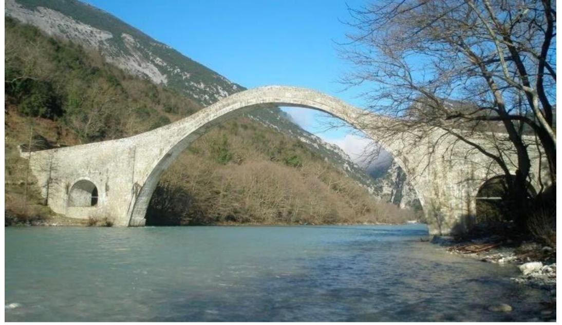
The Plaka Bridge, over Arachthos River, was the largest stone one-arch bridge in Greece and the Balkans, and the third largest one-arch stone bridge in Europe. Its stone arch measured 40 meters and curved majestically over the river, 21 meters above the water. 1866
