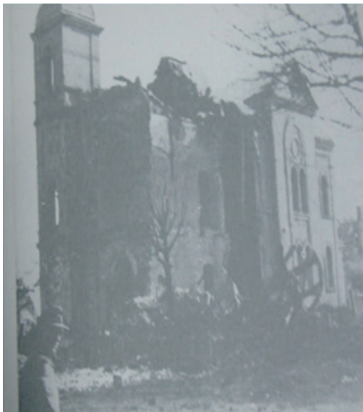
Remains of the synagogue after destruction
